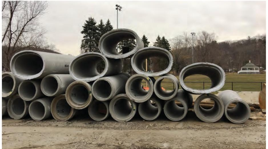
*Replacing more than 1,600 linear feet of cement-lined, ductile iron water main pipes as well as 900-plus feet of connection pipes of varying diameter was a major part of the infrastructure and streetscape plan. They were replaced with 24-inch reinforced concrete piping as well as a new 915-foot twin DIP. (Photo provided)*
